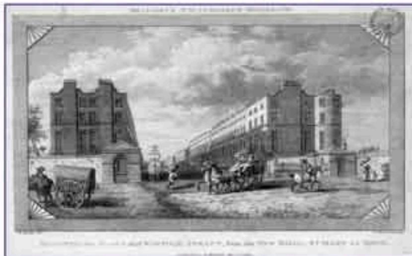
Wimpole Street, 1793 - described in the text accompanying the print as "these piles of building, which unite beauty with convenience, have arisen within these few years, and are at once proofs of the opulence and taste of the Nation" [Ashbridge 120 DEY]
