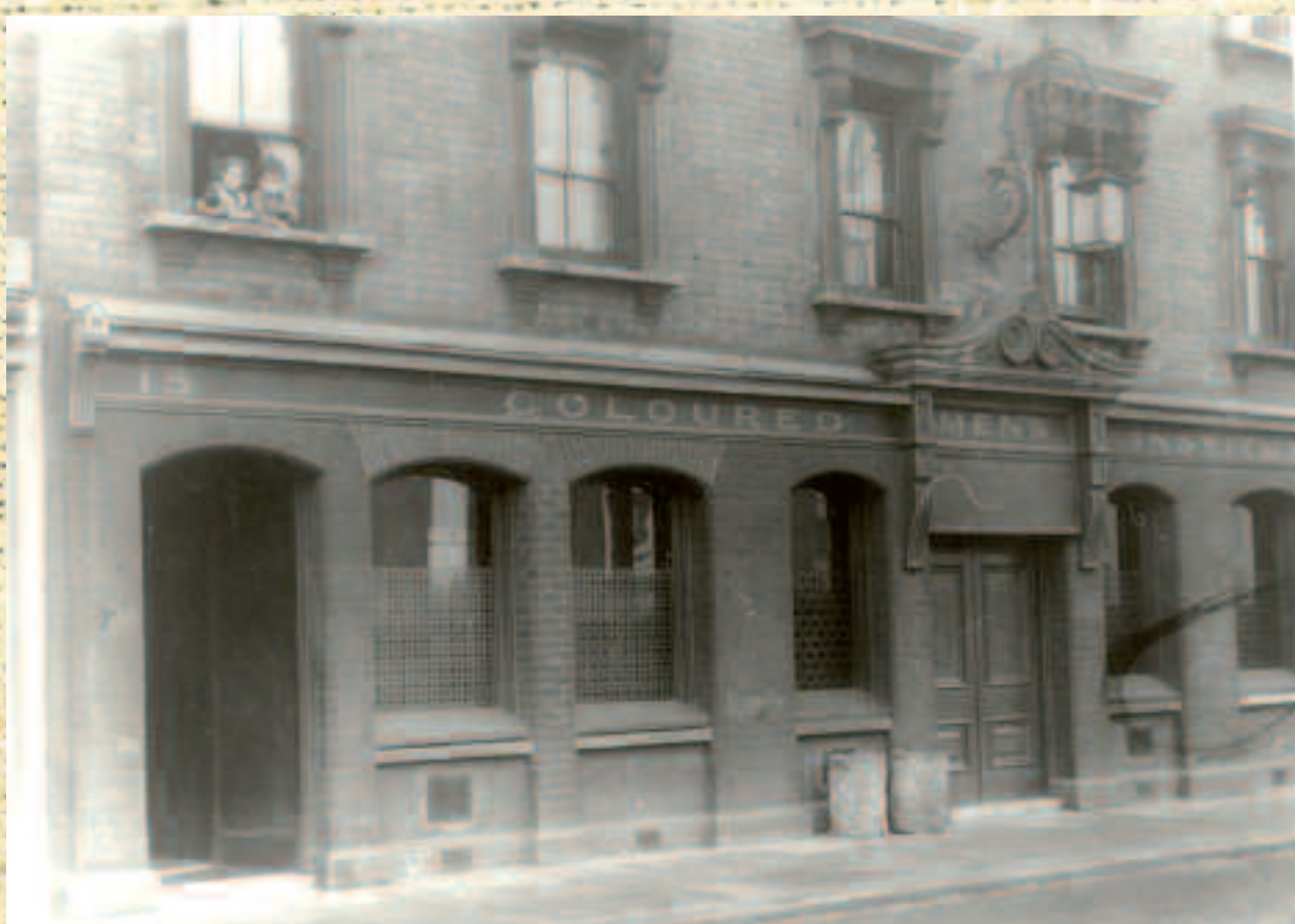
The Coloured Men's Institute, Tidal Basin Road, Canning Town.
