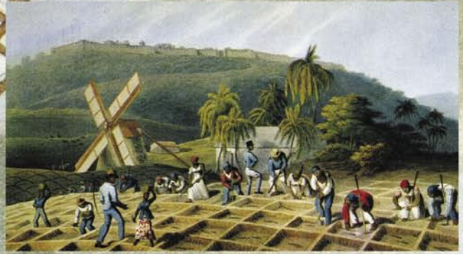
1 Slaves plant cane cuttings and hoe squares of earth
