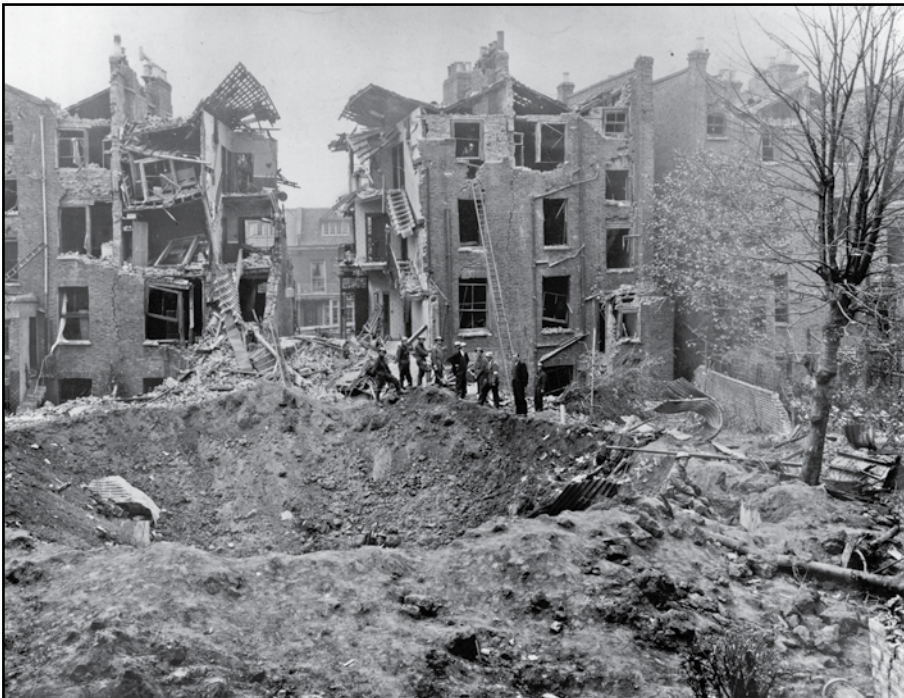
Bomb damage to Ashchurch Grove, 29 September 1940
