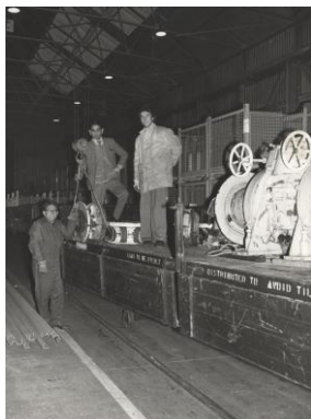
Ahmed Lone (centre), of the Dockyard's Material Management Department, de-equipping HMS Minerva, before a long refit 1976
