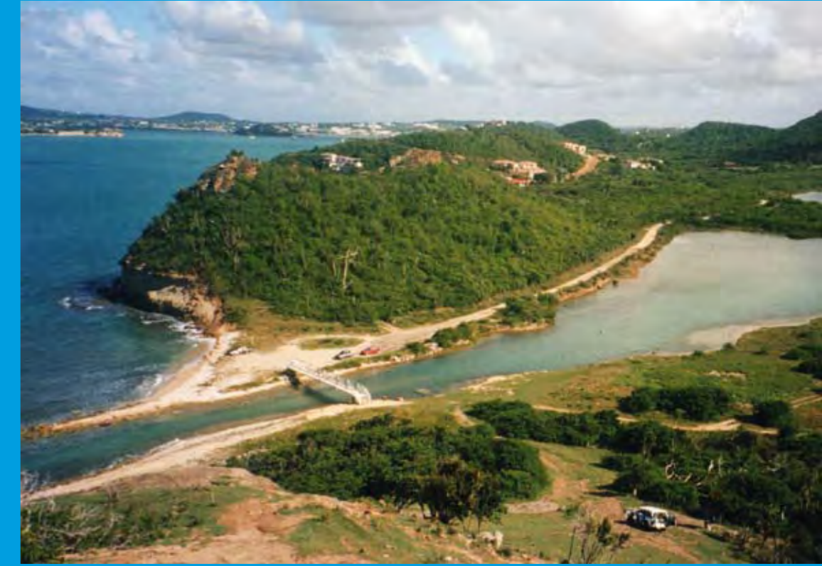
2002 view of the former Codrington plantations on Antigua. Codrington and associated names are commonplace on the island © S Page.
