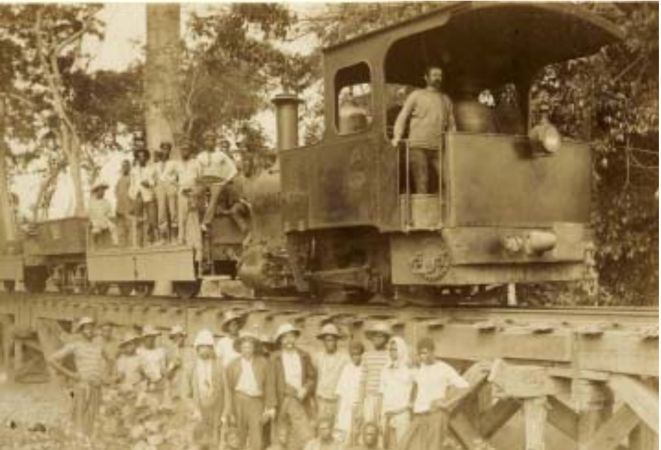
Photo 15: Building the Matadi-Leopoldville railway line. Bas-Congo, 1893-1897
